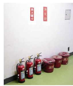
Fig. 5 – Fire extinguishers and fire extinguishing sand
