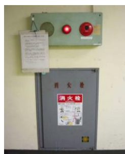
Fig. 4 – Fire alarm and fire hydrant
