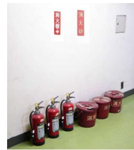
Fig. 5 – Fire extinguishers and fire extinguishing sand
