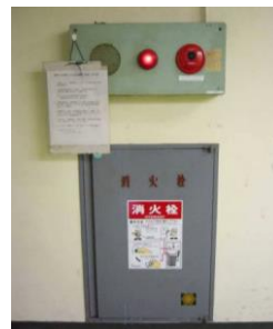
Fig. 4 – Fire alarm and fire hydrant
