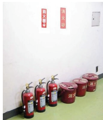
Fig.5. Fire extinguishers and fire extinguishing sand
