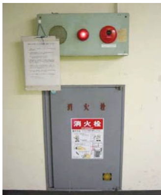
Fig.4. Fire alarm (top) and fire hydrant (below)
