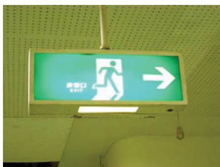
Fig.2. Lights indicating evacuation routes
