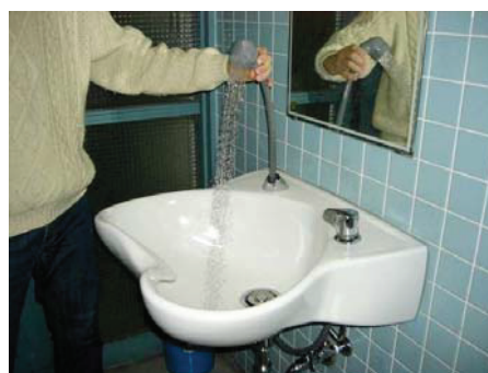
Fig.3. Emergency showers (located in washrooms)
