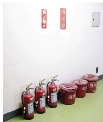
Fig.5. Fire extinguishers and fire extinguishing sand
