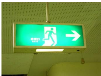
Fig. 4 – Lights indicating evacuation routes
