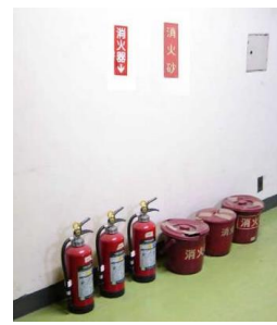
Fig. 7 – Fire extinguishers and fire extinguishing sand
